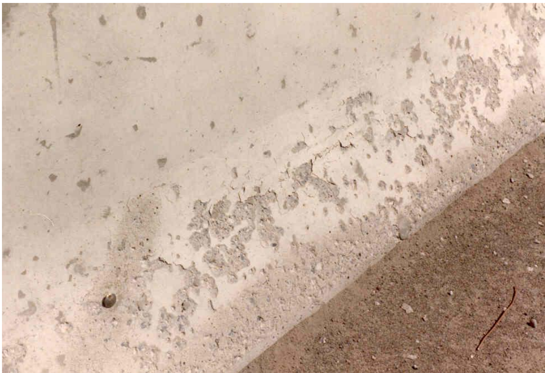
FIGURE 4 Example of Medium Scaling
