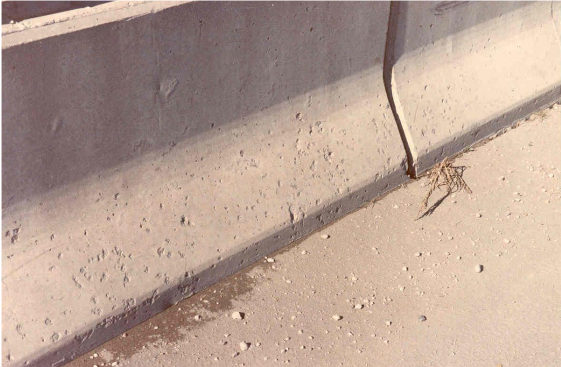
FIGURE 1 Example of Light Scaling
