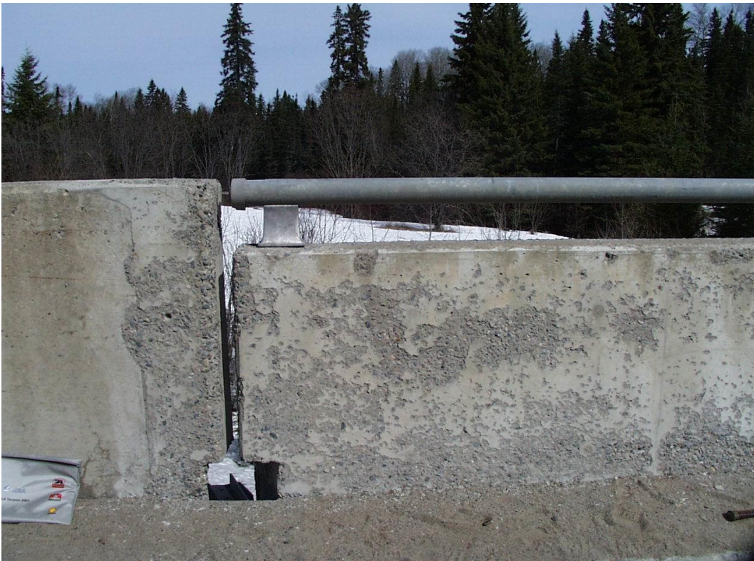
FIGURE 6 Example of Severe Scaling
