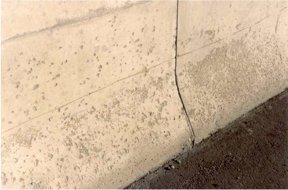
FIGURE 4 Example of Medium Scaling
