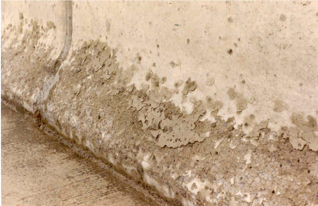
FIGURE 5 Example of Severe Scaling
